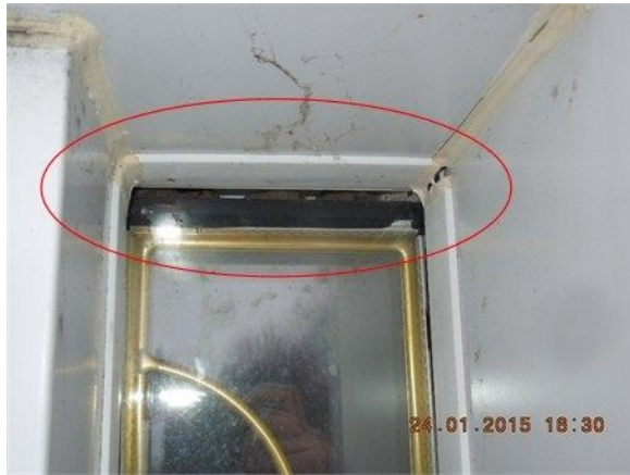
second floor balcony
