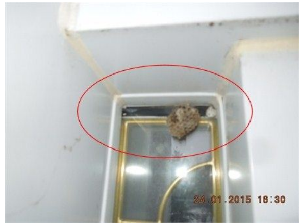
second floor balcony
